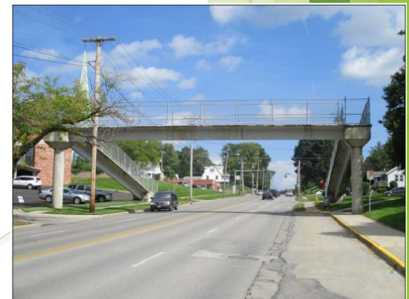
(B2) Overall structure (looking east)
